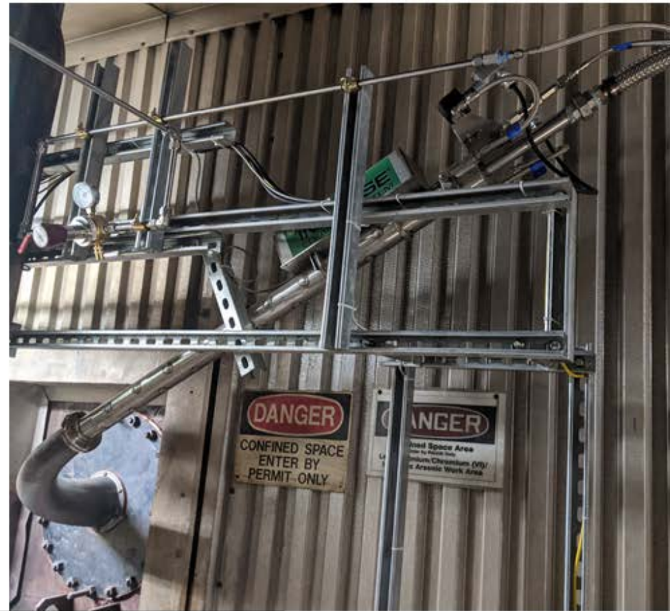
IMPULSE cleaners Installed on North Side of Boiler
