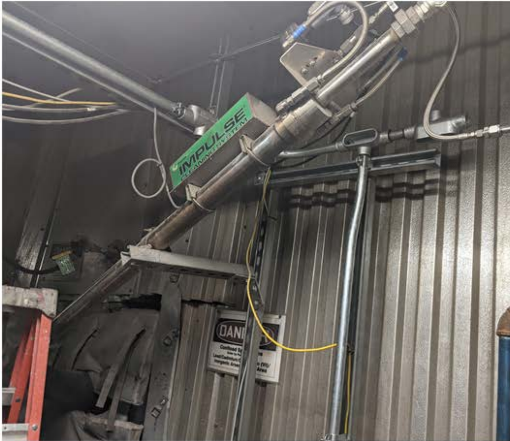
IMPULSE cleaners Installed on North Side of Boiler
